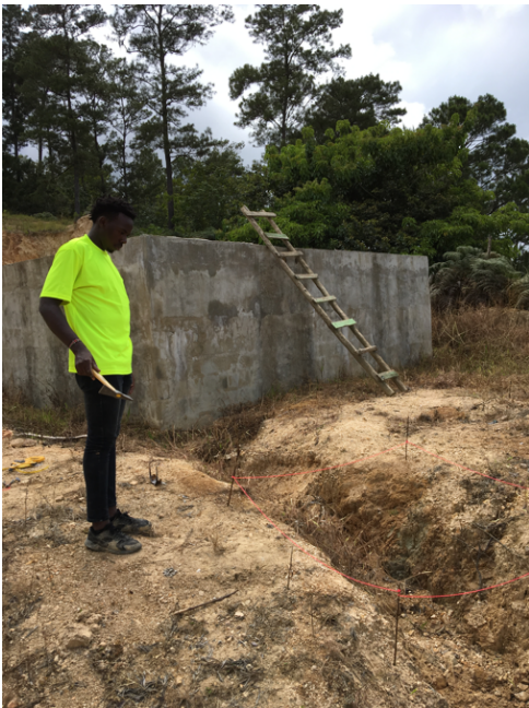
Figure 3-2: (Left) Billy Koech, a member of the project team inspecting the ground in preparation for construction of the tank valve box, with the tank shown in the background. (Right) A Los Sanchez community member, Antonio Cara, with chapter members, mixing concrete in preparation to construct the Alta Gracia valve box.
