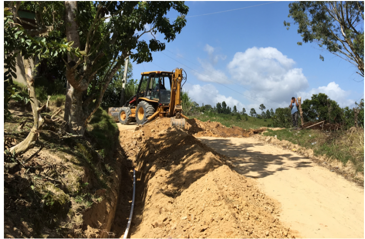
Figure 3-4: (Left) Alan Bidart, a translator and member of the project team, preparing the community agreement in Spanish. (Right) Excavator excavating across the Main Road to connect the 2-in. PVC main line to a house on the opposite side of the road.
