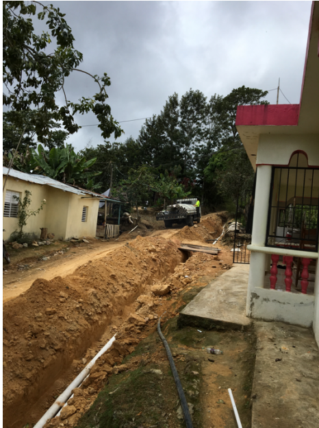
Figure 3-3: (Left) A completed segment of 4-in. PVC pipe with the 2-in. PVC pipe from well to tank visible. (Right) Billy Koech, a member of the project team, laying out the excavation zone for pipe connections into the tank.
