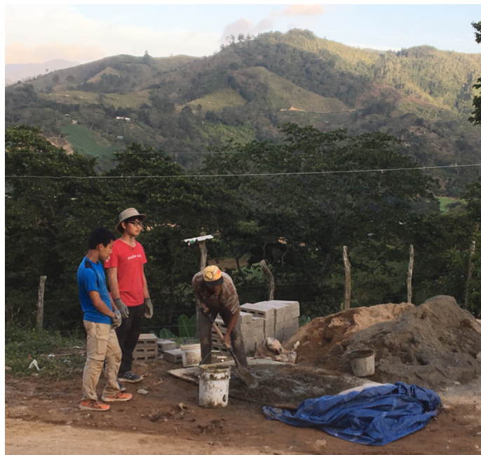
Figure 3-2: (Left) Billy Koech, a member of the project team inspecting the ground in preparation for construction of the tank valve box, with the tank shown in the background. (Right) A Los Sanchez community member, Antonio Cara, with chapter members, mixing concrete in preparation to construct the Alta Gracia valve box.
