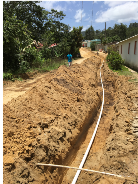
Figure 3-1: (Left) Excavator at a pause in trench-digging, pictured with Saul the operator. (Right) A finished segment of 2-in. PVC pipe laid along the side of the Main Road.
